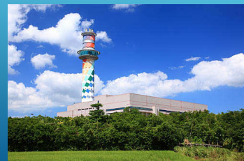
Beitou Refuse Incineration Plant
